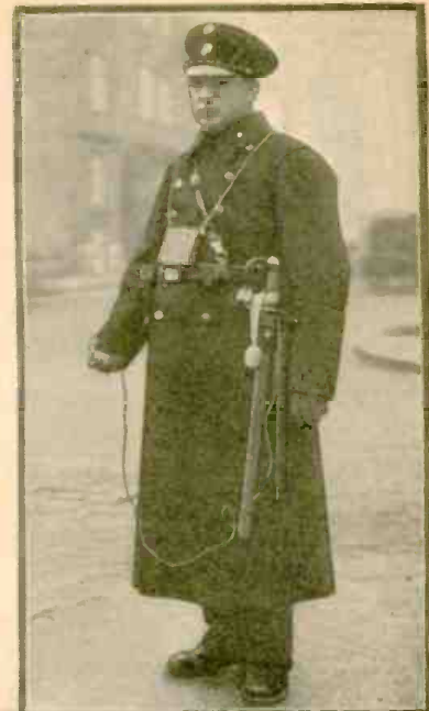
The Vienna policeman we see at right is sending reports to headquarters by means of the portable short-wave transmitter hung on his chest. Left—sending and receiving antennae at Vienna Police Headquarters.
